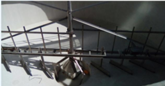
The Tecno Classic system for a lamellar decanter with a diameter of 11 meters.
