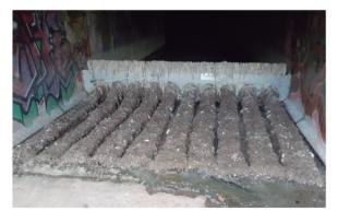
One of the biggest problems encountered when TecnoGrabber® retention meshes are installed in spillways is that they are spaces that are difficult to access and, therefore, they are points that are difficult to control.
