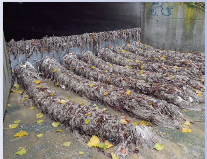
Stainless steel TecnoGrabber® baffle with upper comb
