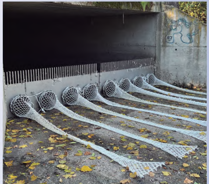
Stainless steel TecnoGrabber® baffle with upper comb
